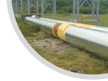
Moulded polyurethanes scales or shells can be used to insulate pipelines **in situ** or as an **alternative** to in situ joints. Two scales are joined around an existing pipeline and are then fixed and **encapsulated** into a cover that can be made of many different materials but mostly by metal or glass reinforced polyester shells. Shells are conveniently used to retrofit old-fashioned mineral wool or foamed cement insulated pipelines.
